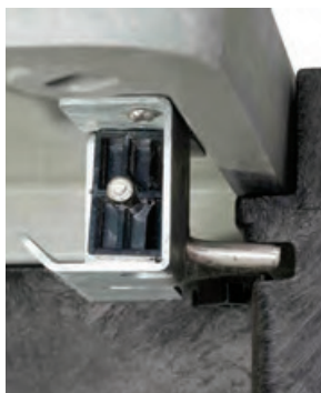
L-Bolt Security System (SHIELD Cover Shown)
