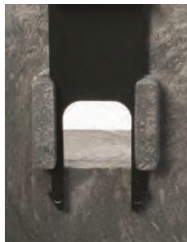
Winterized Cable Drop Side
